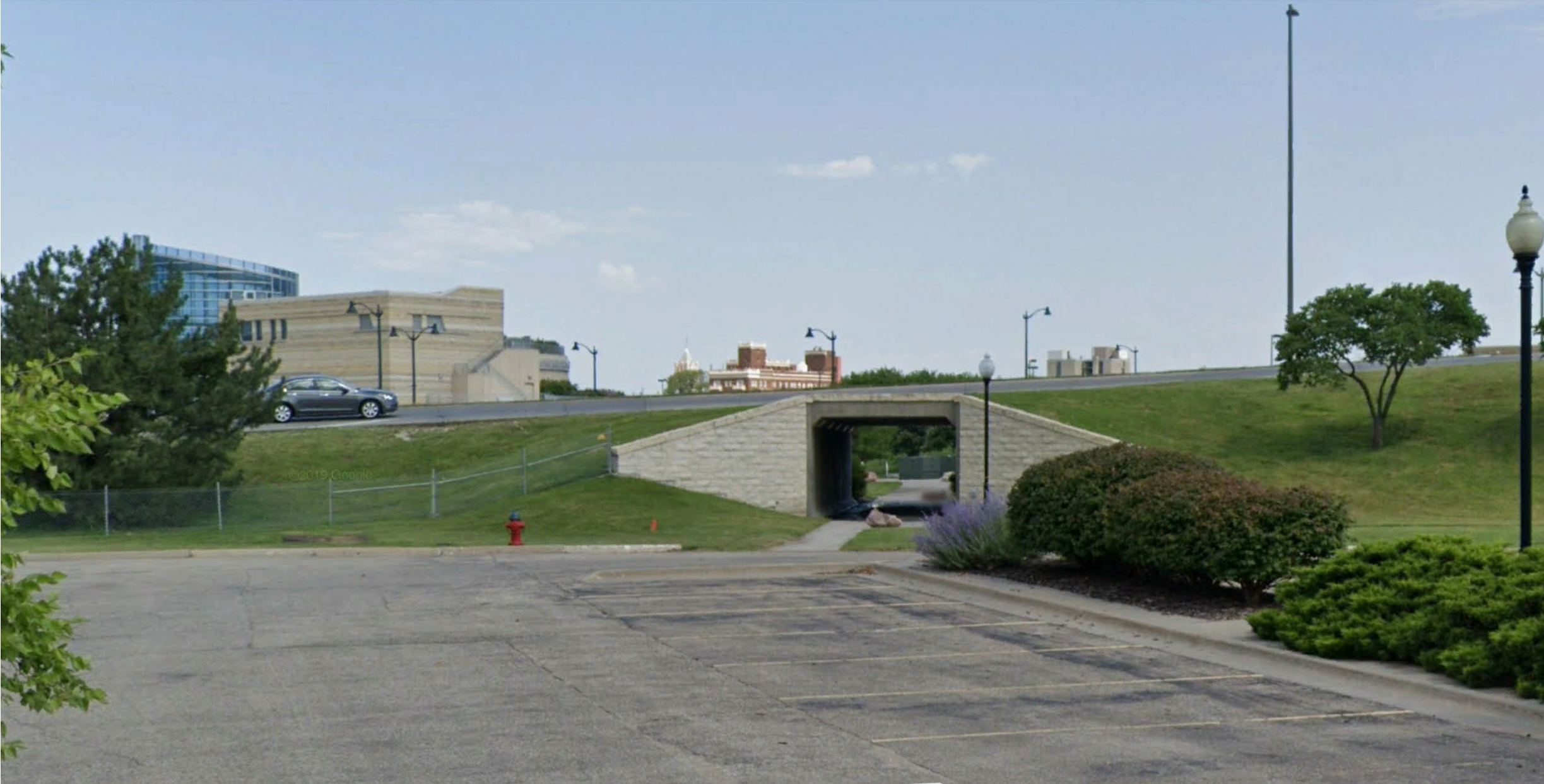
Example: Union Depot Tunnel
